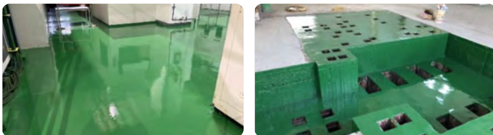
Figure: New Plant Construction Featuring Epoxy Floor Coatings Made from Recycled Silicon
